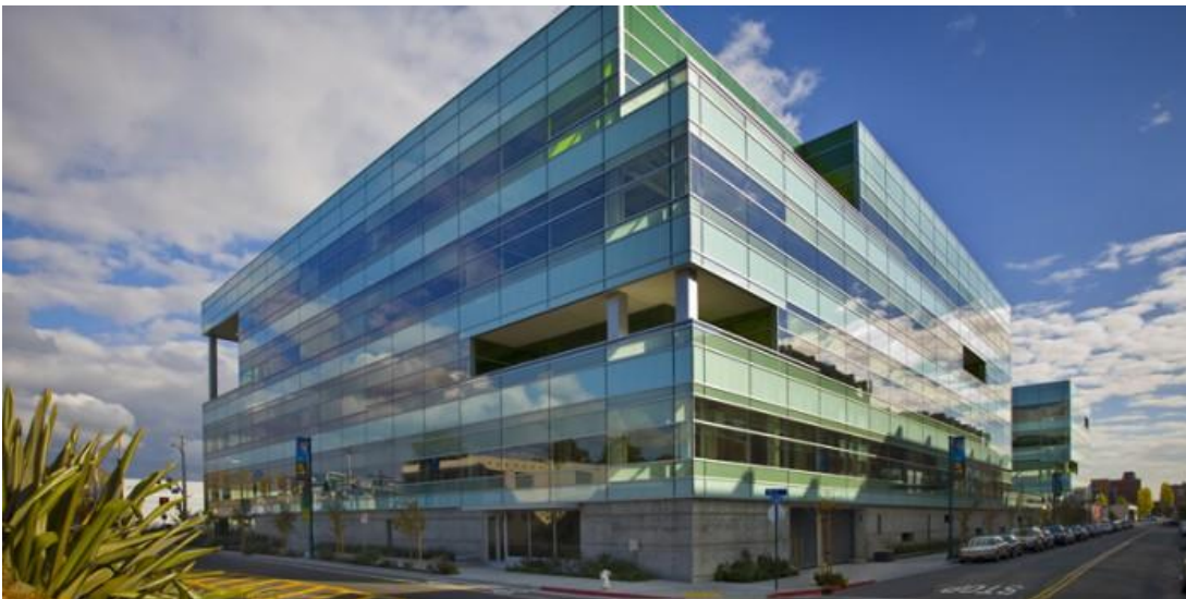
Joint BioEnergy Institute, CA
